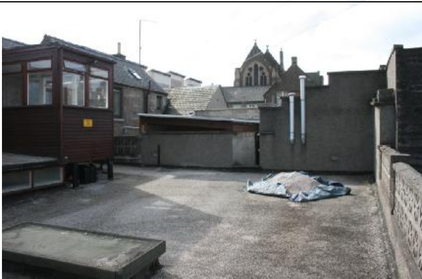
The extended basement roof to the rear of the flats
