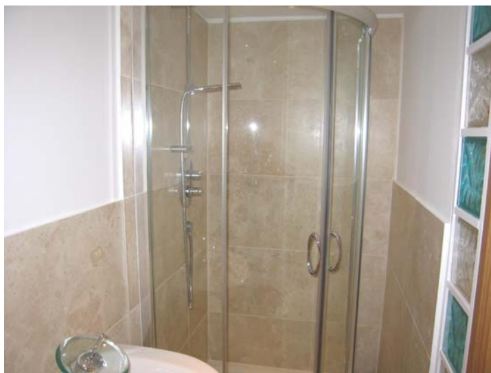
Ground Floor Shower Room
